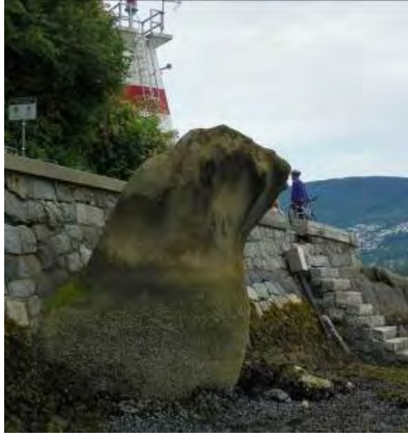
Figure 28: Suntz in badly eroded condition (2013)
